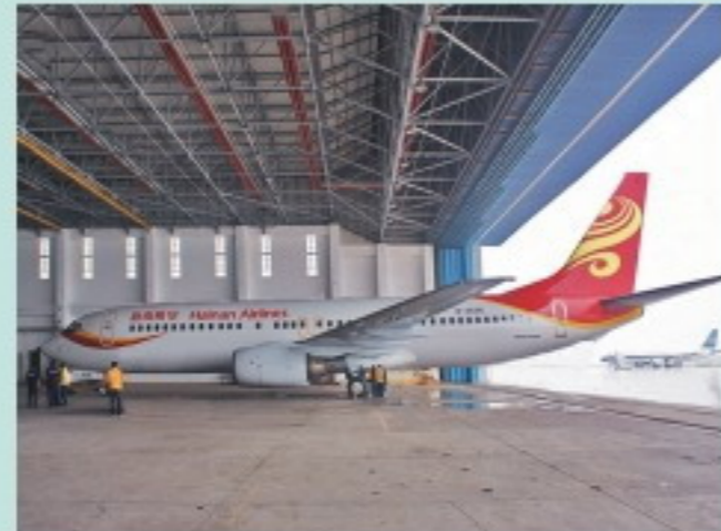
Aircraft Maintenance Plant
